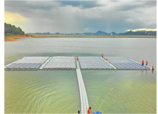
108 kWp Floating Solar Sg. Labu (Research Project)
